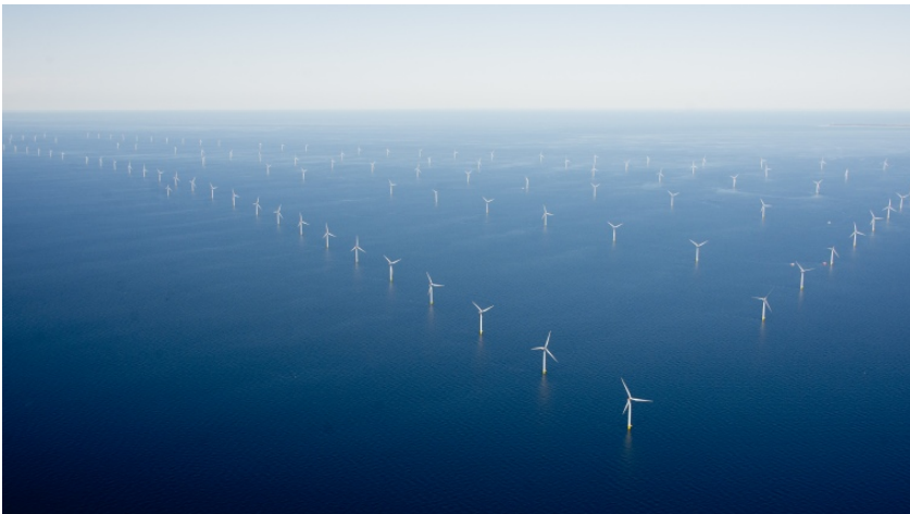
Figure 2.1: The Danish wind turbine farm Anholt , the third largest wind turbine farm in the world.
