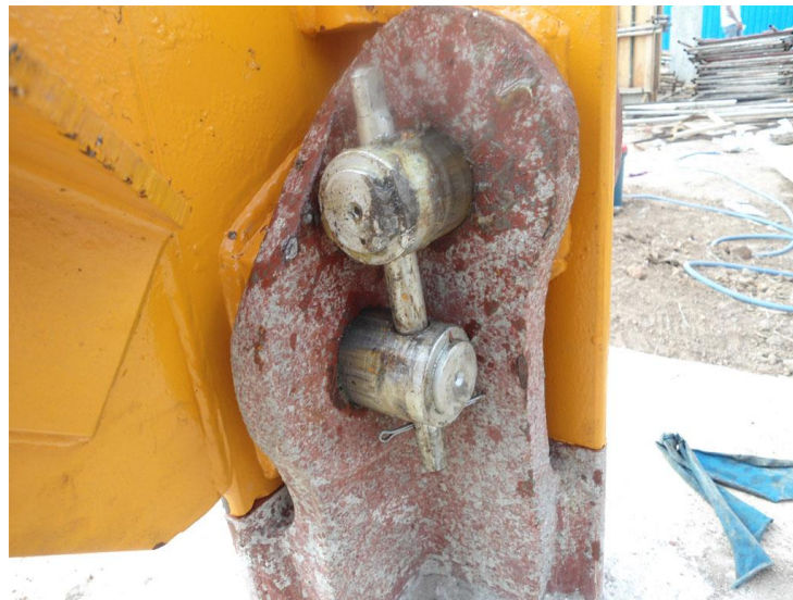
Figure 4: Tower crane foundation connection with pins [7]
