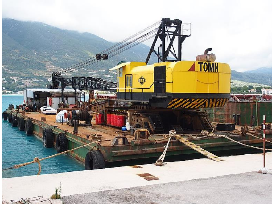
Figure 24: TOMH crane Lima [27]
