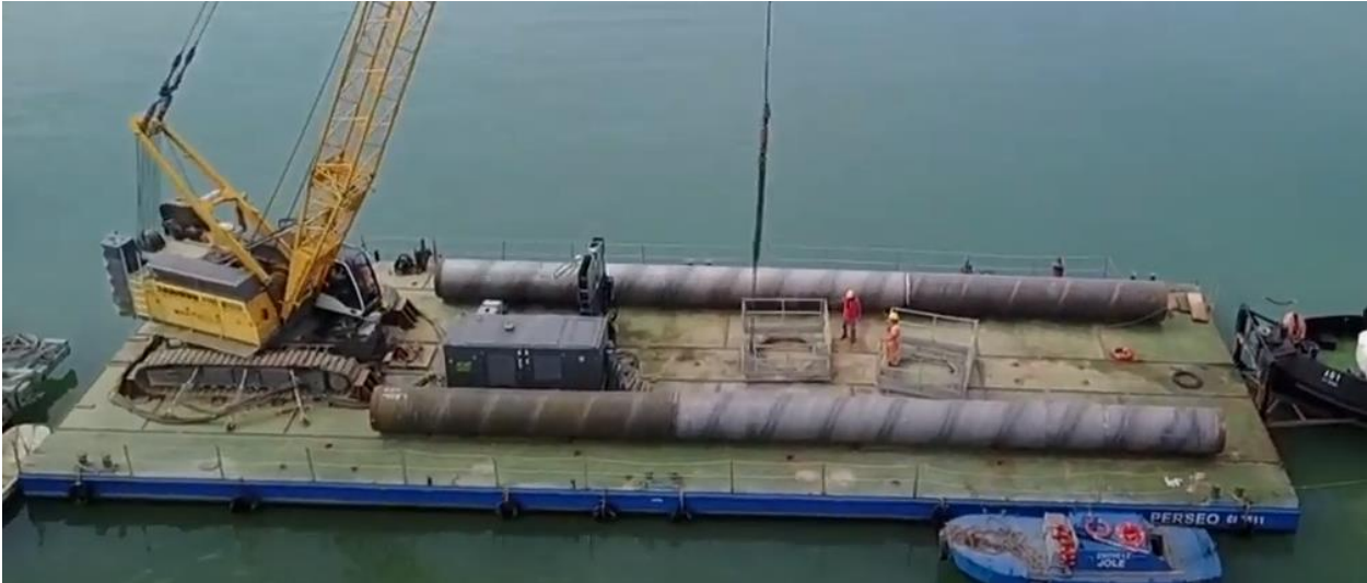
Figure 22: Liebherr crane on pontoon [25]
