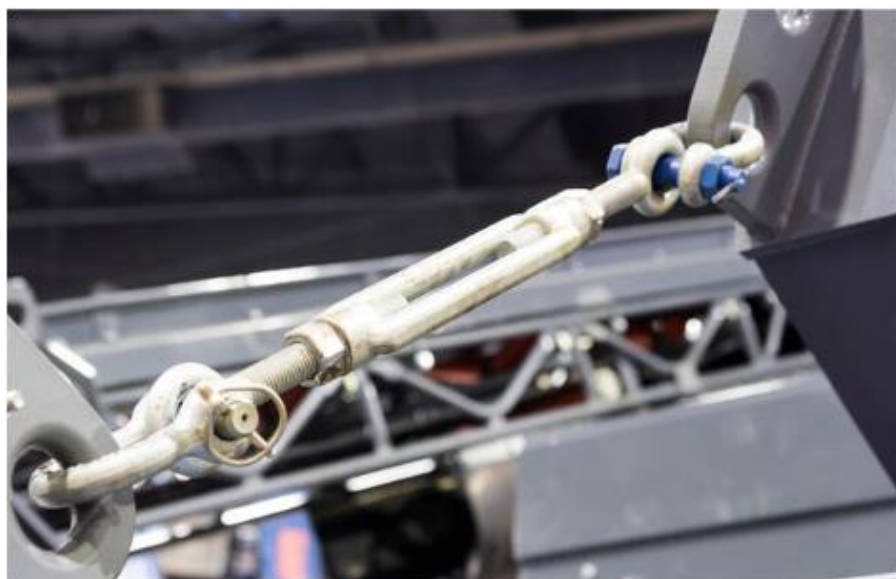
Figure 83: Turnbuckle jaw to lashing eye connection
