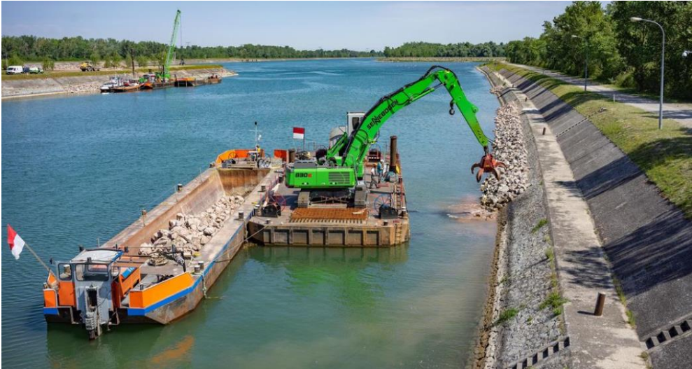
Figure 2: A land crane operating on a floating pontoon [3]
