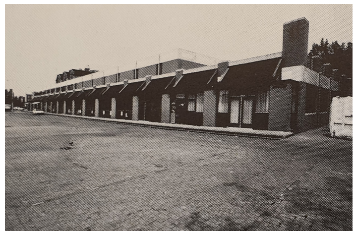
Figure 5.5. Pier 80, South facade connected to the square. (Bulthuis, 1986).
