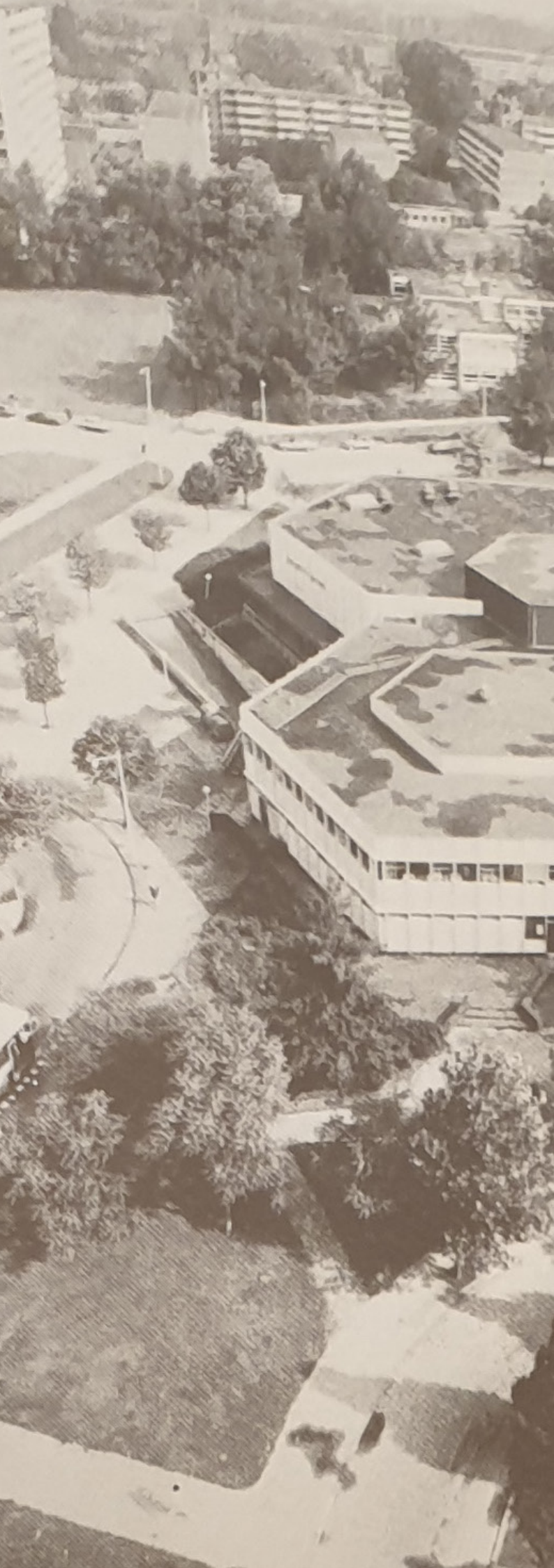
Community centre De Klimmende Bever (Bulthuis, 1986, 75).
