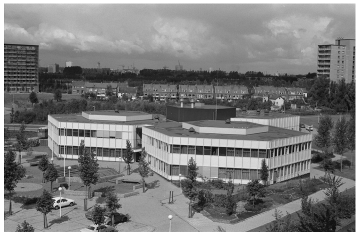
Figure 4.10. Photo of De Klimmende Bever. The specially designed outside space is visible in front of the entrance. (Groeneveld, 1973b, Stadsarchief Rotterdam).
