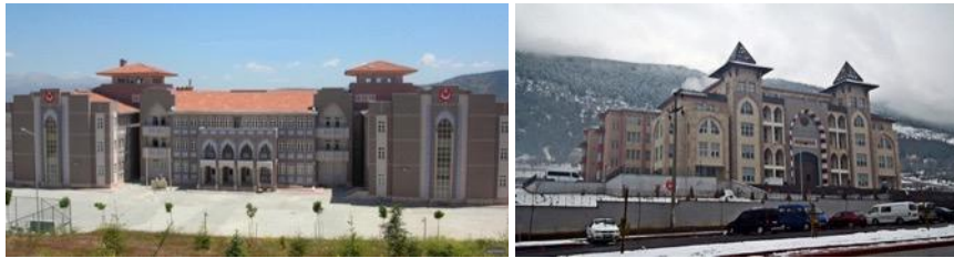
Figure 0.1. A school in Isparta on the left and the courthouse of Kahramanmaraş on the right, both of which have been built in an Ottoman-Seljuk revivalist style. Source: www.moblogankara.org
