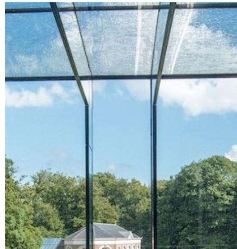
(b) Detail of fin to facade and roof connection. Photo by [64].
