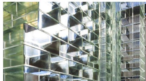
Figure 2.4: Facade made of cast glass bricks at the P.C. Hooftstraat in Amsterdam. Photos by [4]
