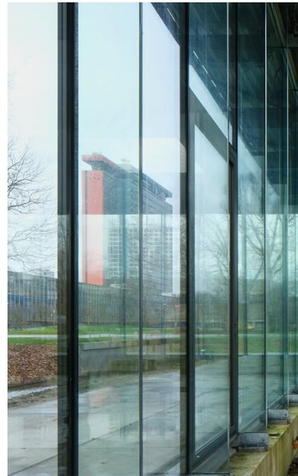
Figure E.2: Fin-facade connection with a 2 component structural silicone sealant.
