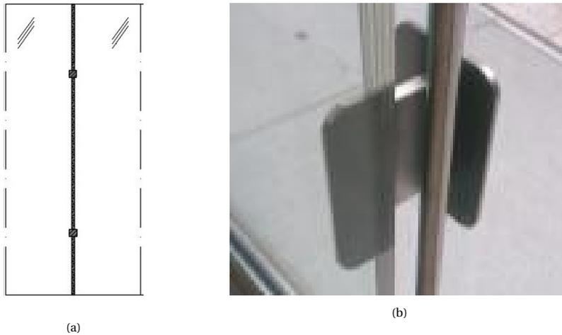
Figure E.8: An embedded connection to connect the facade and fin.
