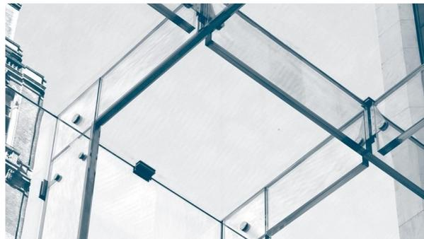
Figure 4.14: The bolted frame connection can be found in the left corner.[23]
