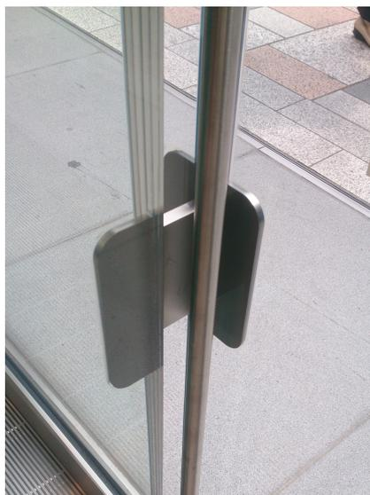
Figure 4.19: Titanium embedded connection in the Apple Store at the Omotesando, Tokyo, Japan. Photo by author.
