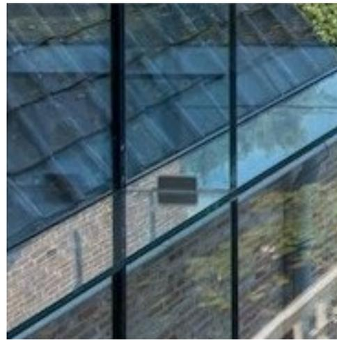
(b) At every crossing of a beam and fin in the facade, an embedded connection is applied. Photo by [64].
