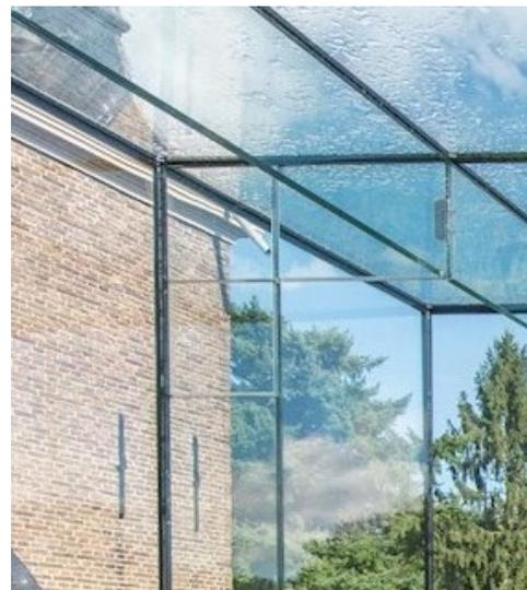
(b) At every corner, an overlap joint has been applied, which connects the fins and beams. Also in the facade this connection is applied horizontally. Use is made of "Delo-Photobond 4468", which is a UV-curing adhesive. Photo by [64].
