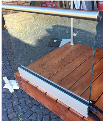
Figure 4.22: An example of a line support with an u-profile bearing. This variant uses a dry connection which is ideal for deconstruction. [27]
