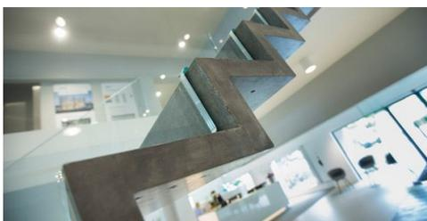
(a) Epoxy has been applied to create a local stiff point to connect the concrete and glass. Photo by [139]
