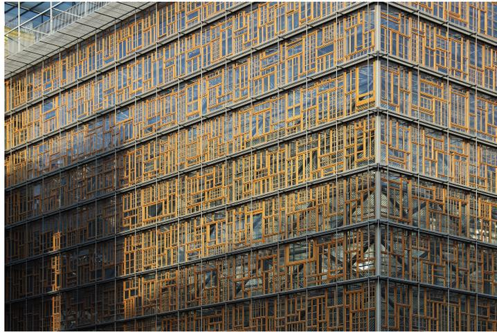
Figure 3.2: Old timber frames are reused in the facade of the European Union Headquarters in Brussels. [9]
