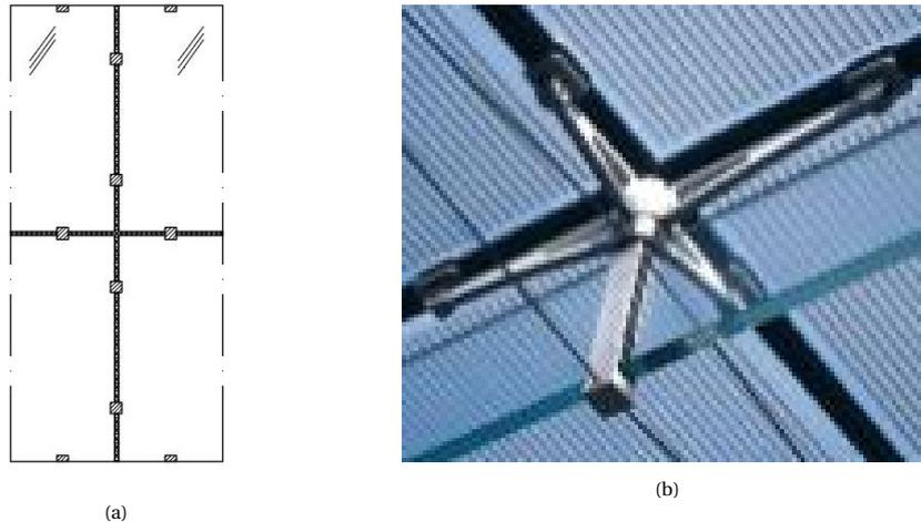
Figure E.7: A clamped spider connection to connect the facade and fin.
