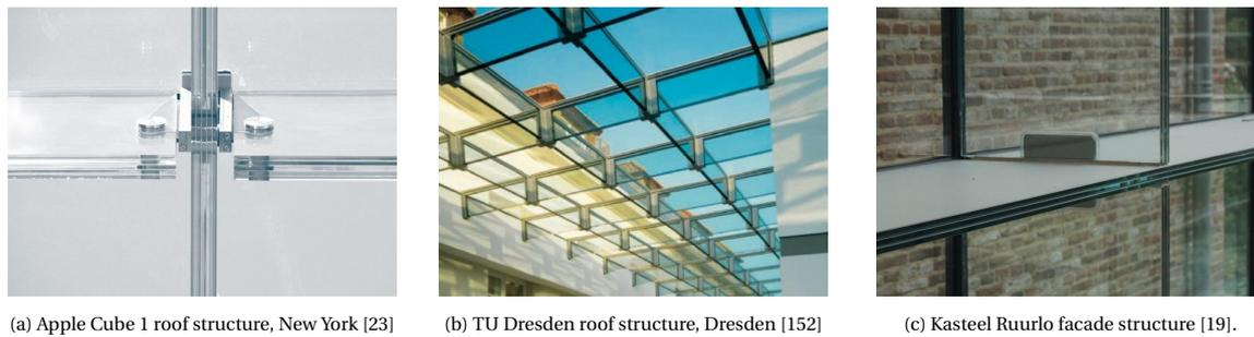
Figure 8.5: Fins are required in design for both facades and result in the roof grid.
