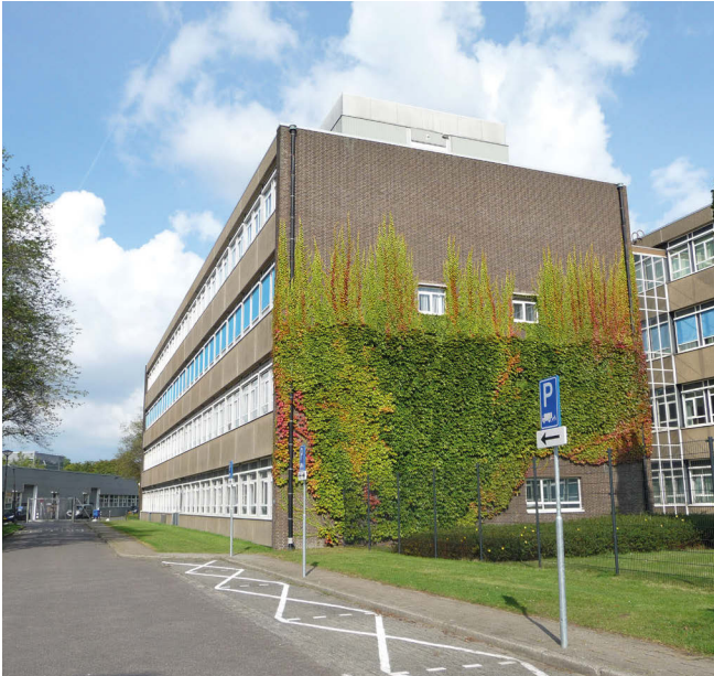
Photo 1. Front view of Former Verbindingschool. Source: J.J.M. Aling (2017)
