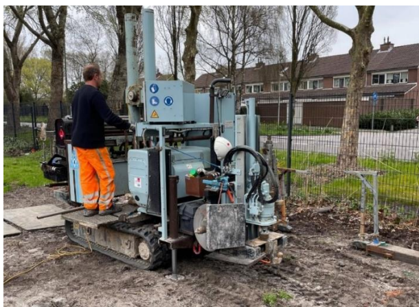
Figure 23. CPT rig with SCPTU modifications.
