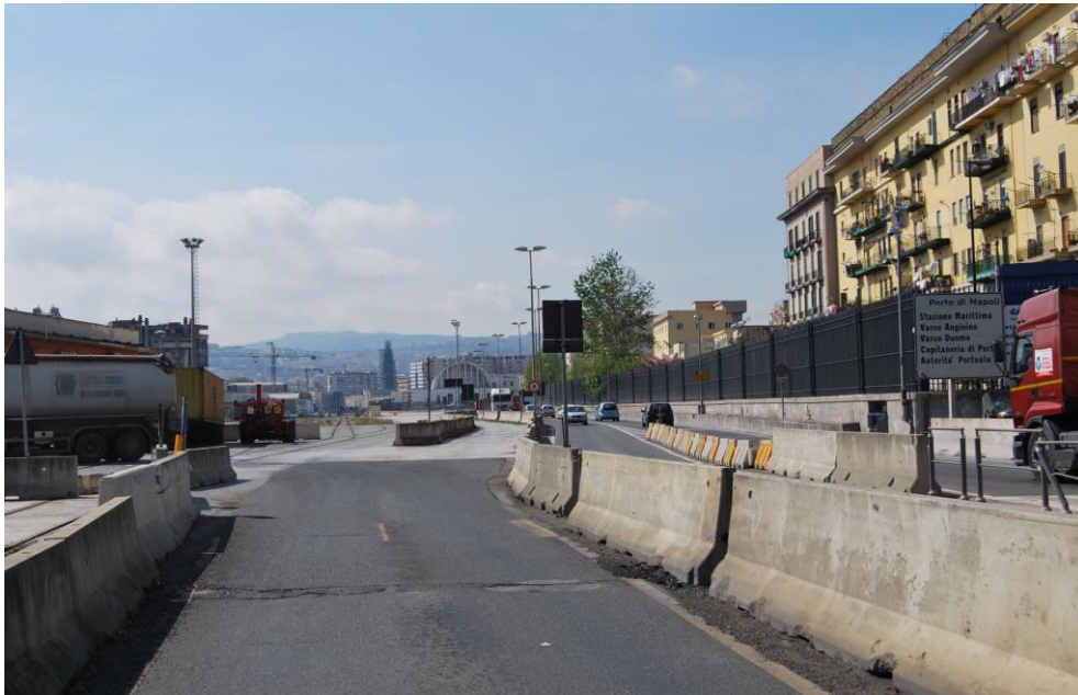
Fig. 1 – Barriers which separates the port from the city, East Naples, 2018
