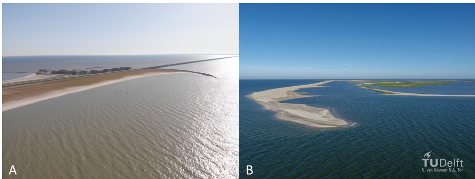
Figure 1.2: Drone images of the Houtribdijk with the FL67 measurement stations (A, March 2020, by Bureau Start the Future commissioned by Rijkswaterstaat) and the southwestern side and spit of the Marker Wadden (B, April 2022, by Niels van Kouwen and Anne Ton)
