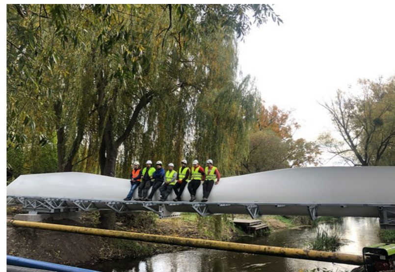
Figure 24: The first pedestrian bridge made from WTBs designed and installed by Poland-based Anmet (Mason, 2021)
