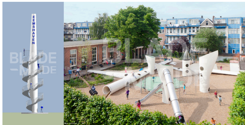
Figure 22: A lookout tower with a WTB as the main support structure (left) and a playground made from WTB sections (right) designed by Superuse spin-off Blade-made (Blade-made, n.d.).
