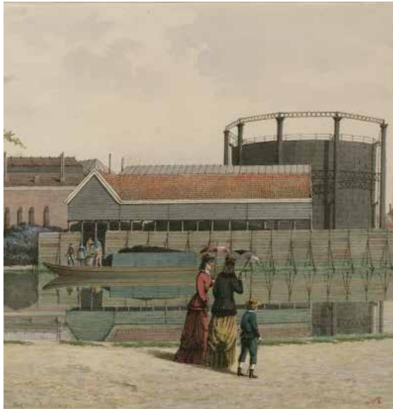
Gas factory on the site in the XIX th century
