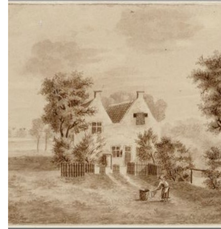
1810 - Stronghold Nieuwkerk after demolition of the mill
