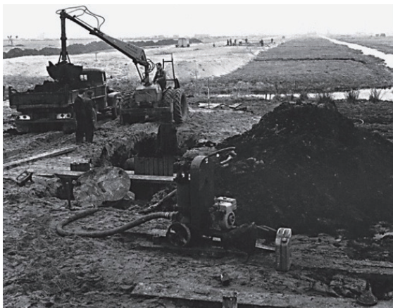
Figure 1.1, showing Soil Improvement by filling of land. Source: De Ingenieur
