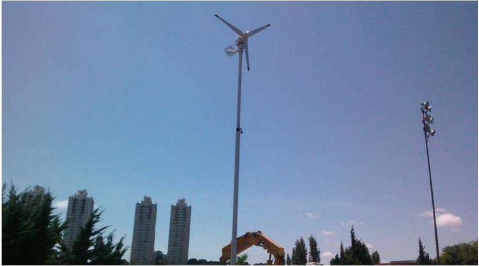
Figure 10. Final aspect of Wind Turbine Installed
