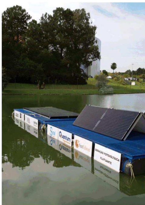
Figure 4. Ferry Solar Photovoltaic Panels Details
