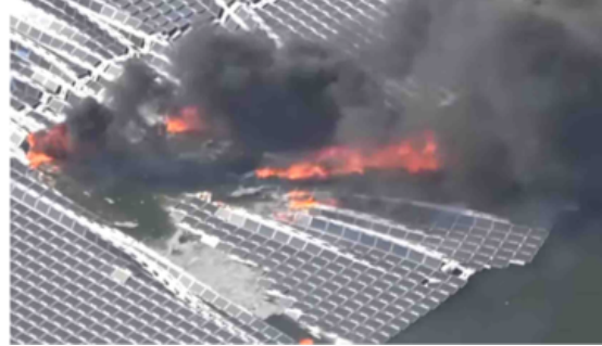
Figure 1.9: Fire on Yamakura Dam FPV [54]
