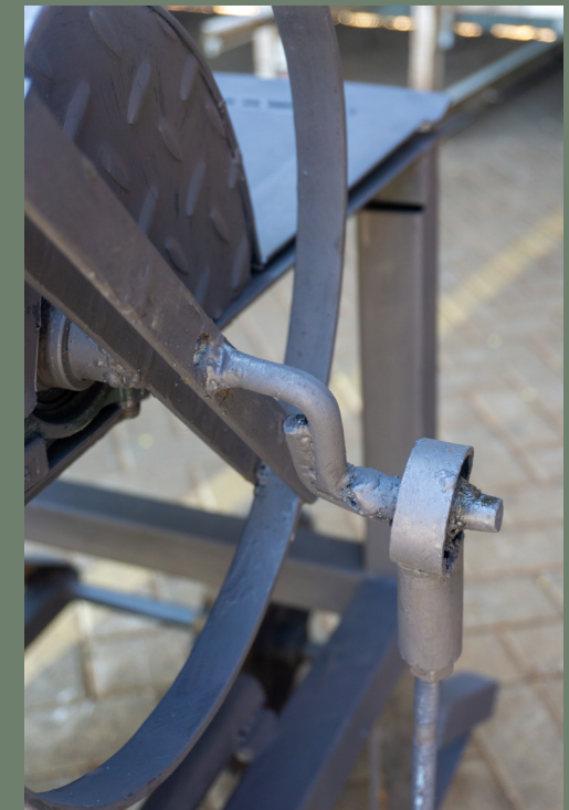
Image 39. Pulley connection. Photograph by Marte Lanning.
