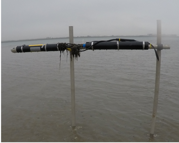
Figure 4.4: ADCP frame with external battery canister. Taken on 03.02.2021
