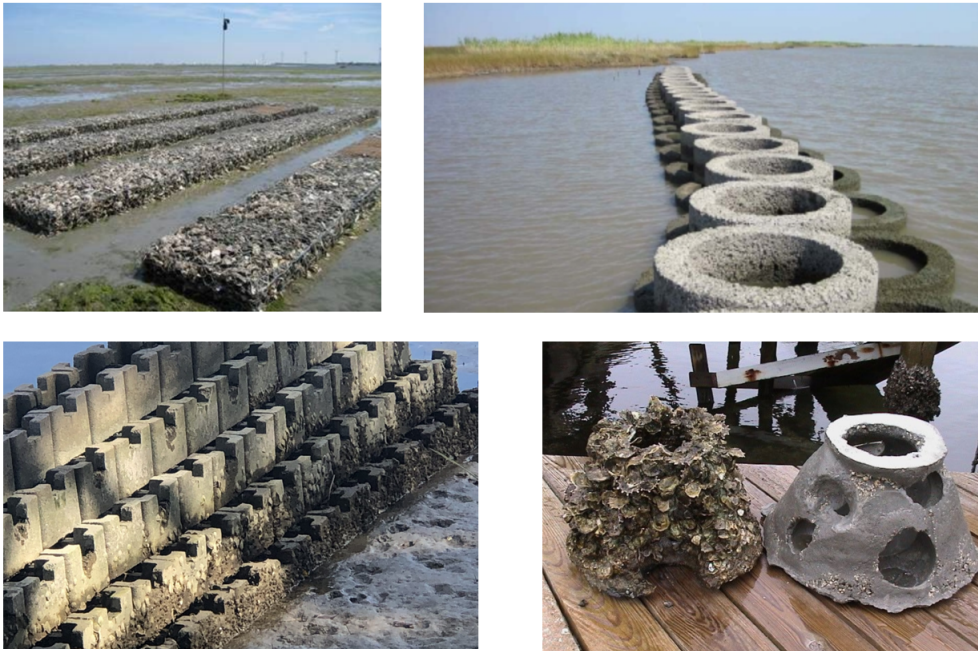
Figure 2.2: Different artificial oyster reef structures in practice. tl: shell gabions used in the Netherlands (ecoshape.org), tr: OysterBreak™ (Wayfarer Environmental Technologies), bl: The Oyster Castle@alliedconcrete.com), br: Oyster Reef Ball (reefinnovations.com)
