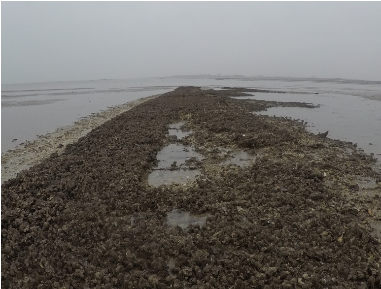
Figure 1.2: Artificial oyster reef built on an intertidal flat. Photo taken during emergence at low tide.
