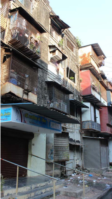
BDD Chawls / Encroachment
