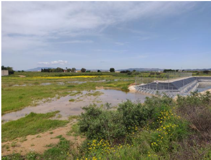
Figure 1.5: Dry river location B.
