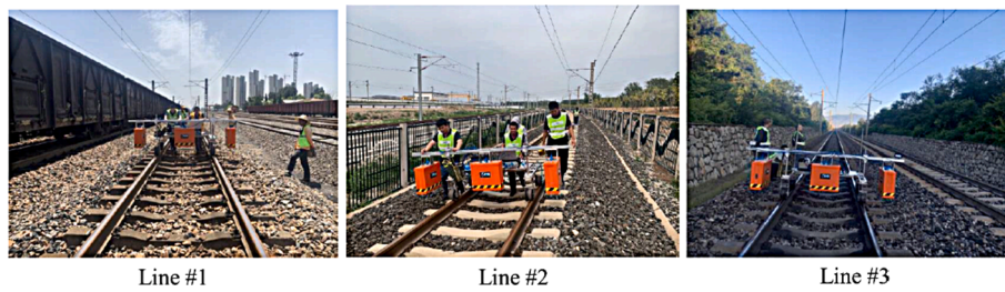
Fig. 7. Three examples of railway lines inspected by GPR.
