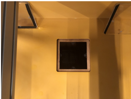
Figure B.10: Hatch with transparent lid at top of the picture. Two of these hatches located at floater top, two at bottom
