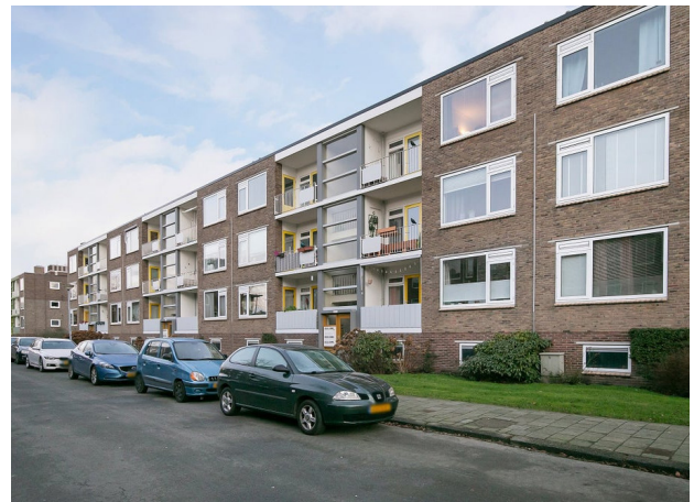
Figure 21. Typical portico apartment flat (portiekflat)
