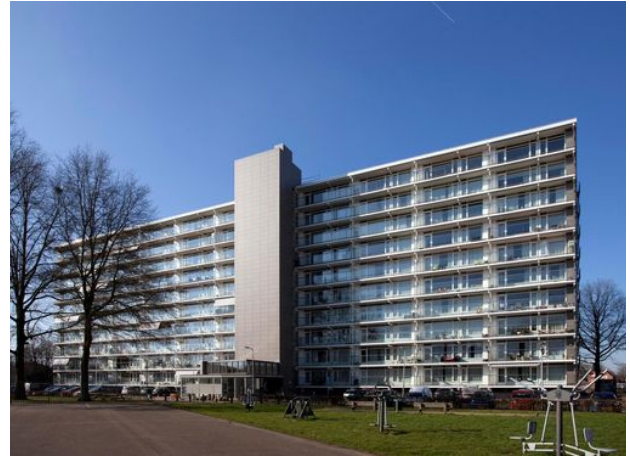
Figure 20. Typical gallery apartment flat
