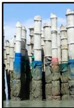
(a) Vertical poles, packed in fiber as protection against ship worm.
