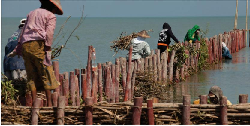
Figure 1.6: Construction of a permeable structure consisting of brushwood (EcoShape, 2018).
