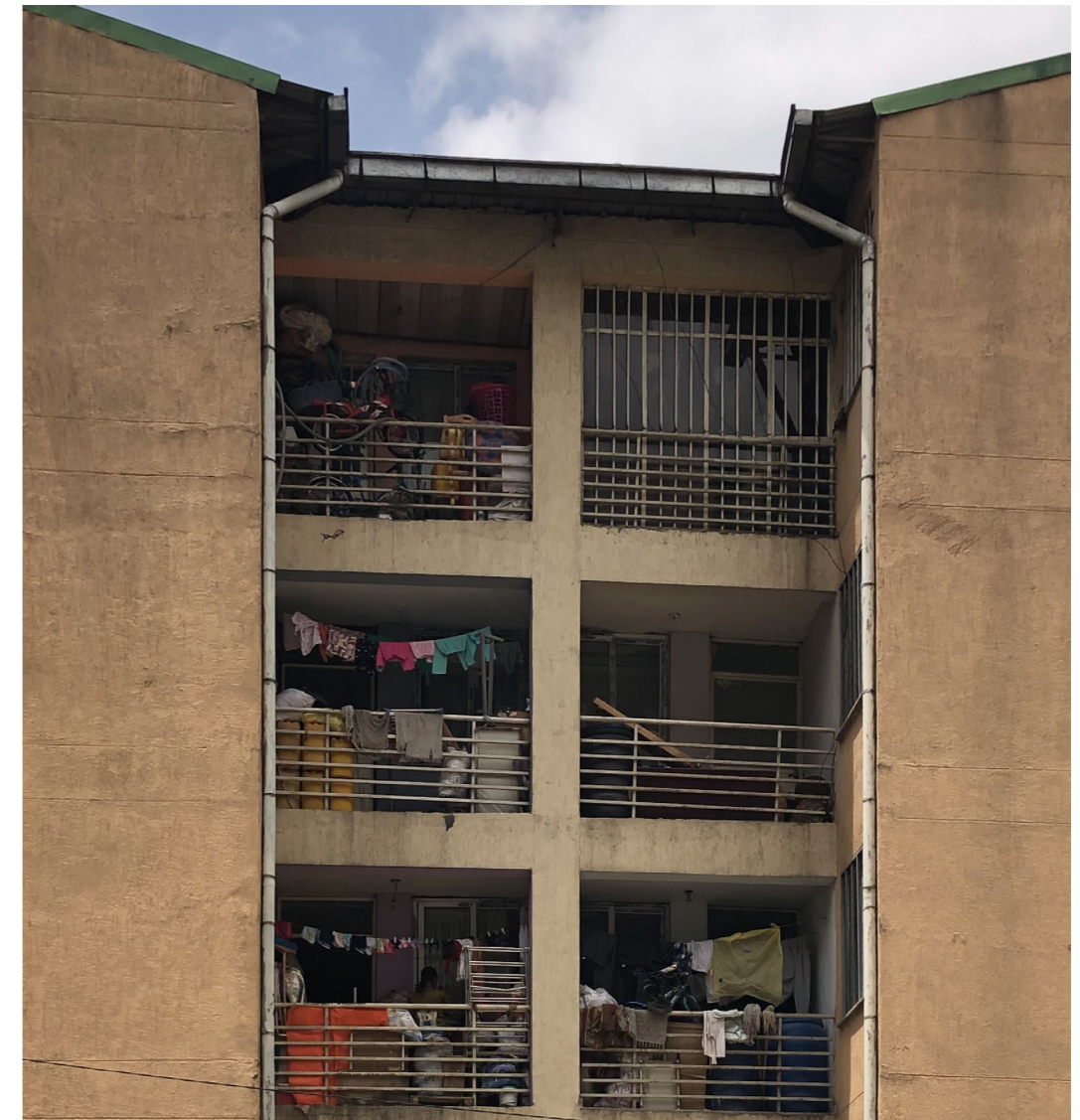
Figure 9: Lideta Condominium loggias showing how the space is used as storage space. Source: Author
