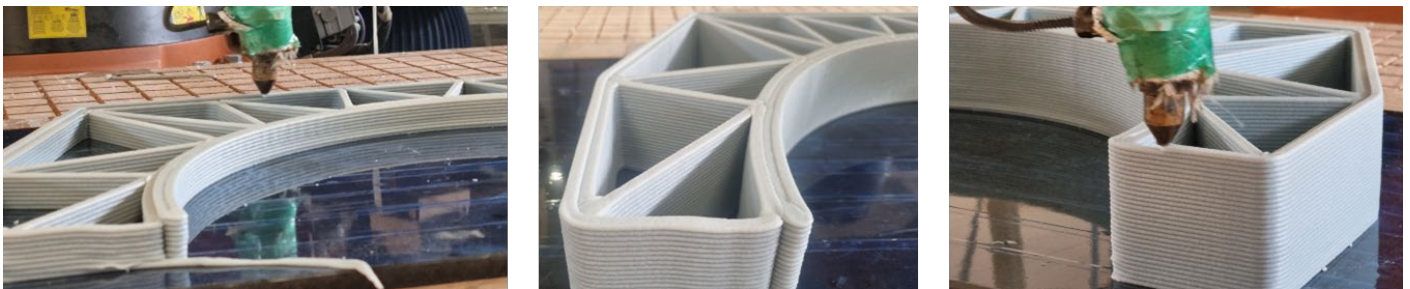
Figure 9-12 Printing process by extrusion layer by layer of the arch elements
