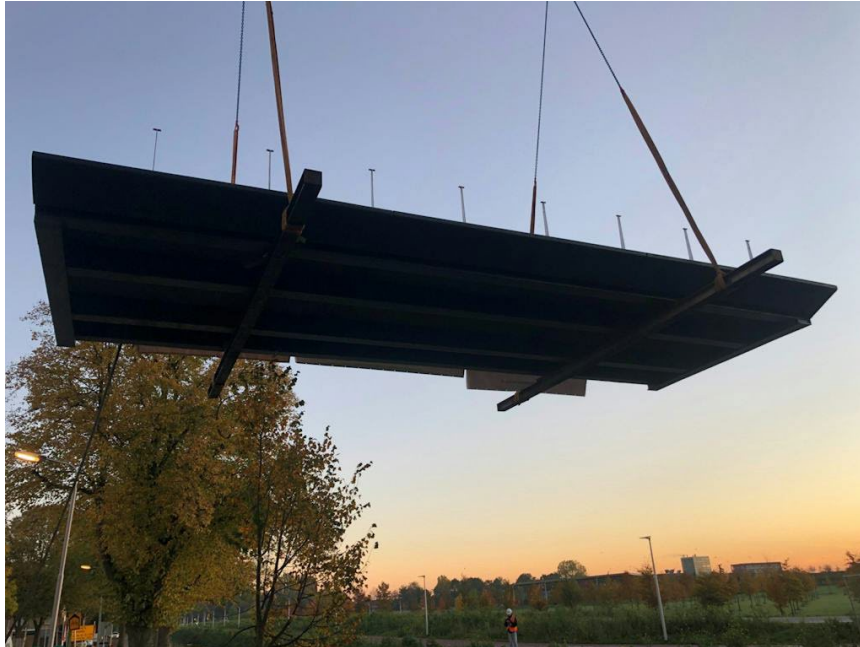
Figure 2-6 3D printed bridge with recycled plastics in Lansingerland [12]
