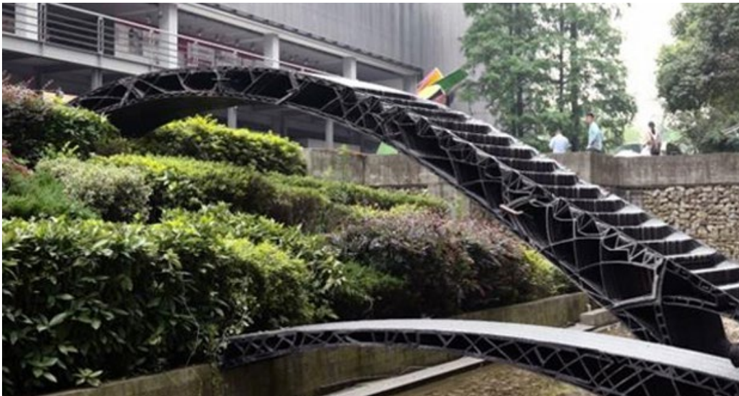
Figure 2-5 The two 3D printed pedestrian bridges in Shanghai [11]
