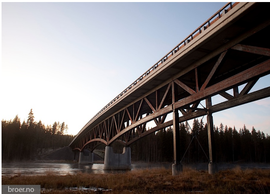
(c) Kjøllsæter Bridge
