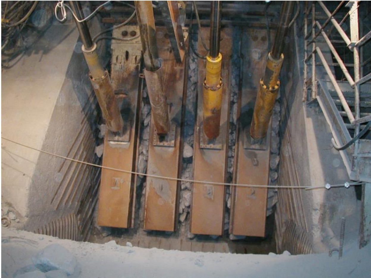
Figure 10 Press gates controlling the material flow in the bottom of the ore pass
