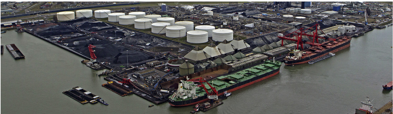
Fig. 8. St Laurens haven terminal aerial view (Image courtesy of EBS BV).
