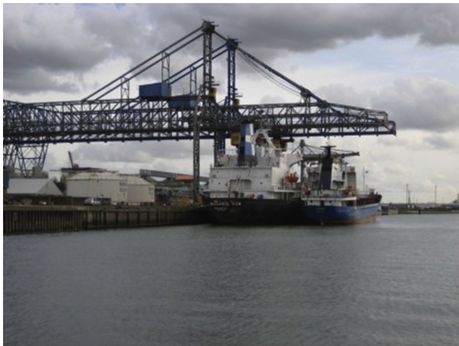
Fig. 13. Direct transshipment operation (Image courtesy of RBT BV).
