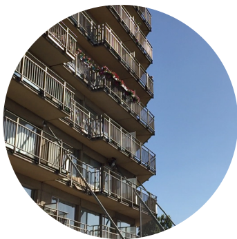
03. Les Goujons - a social building falling apart in every aspect
