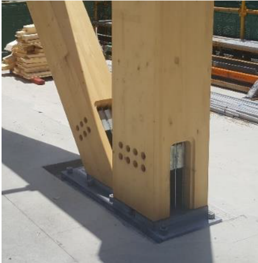
(C) Connection detail (bracing) [33]
