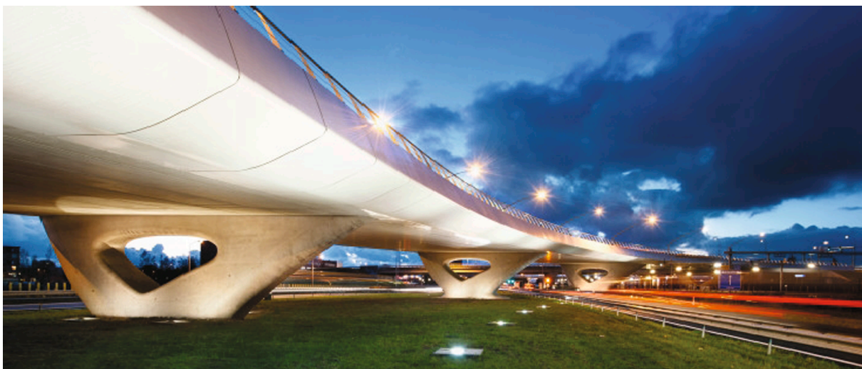
Fig. 1. Fly-over Waarderpolder bridge in Netherland with FRP edge elements [10]. A single column fitting image.
