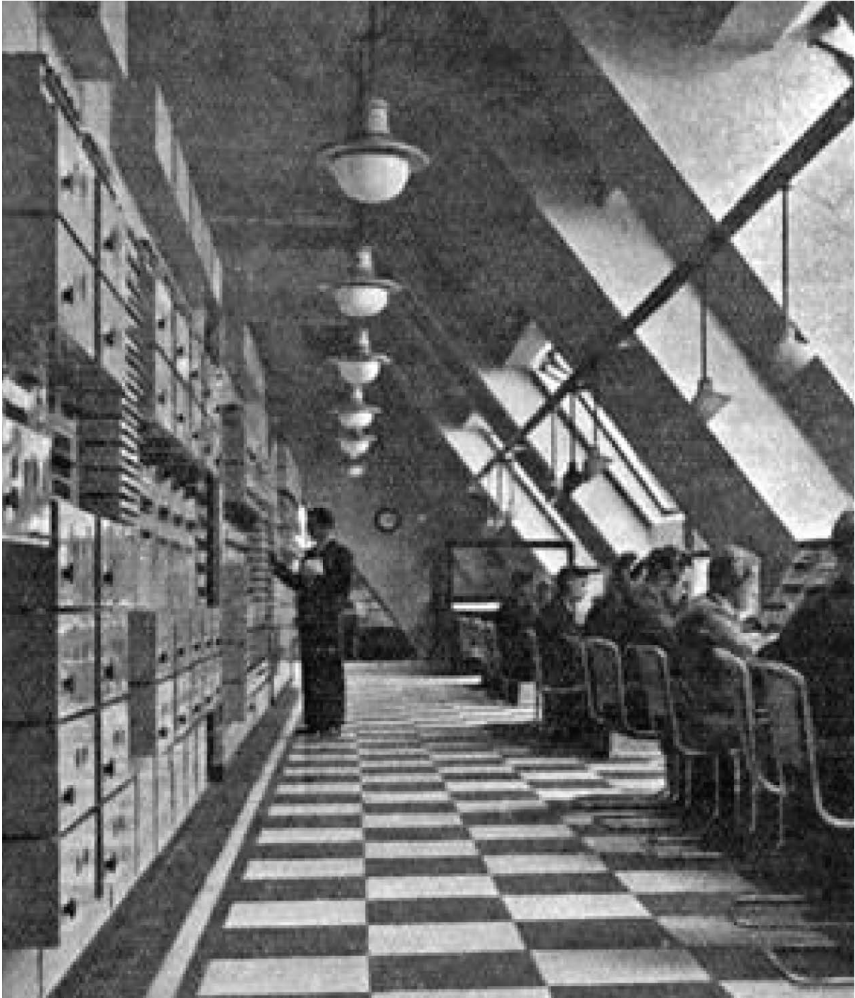
The BBC Broadcast House, Radio Station, 1932. The room is organised around the processes of the technology itself. _C19
