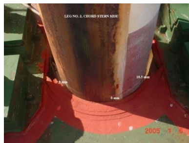
Figure 4-8 Guide plate and leg chord
