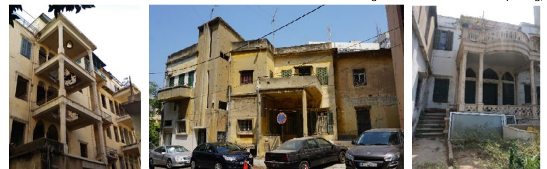
Figure 3.7: Abandoned housing in Mar Mikhael (NAHNOO, 2020)
