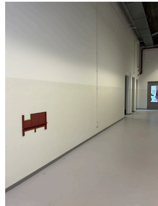
Fig. 29. a lost facade in the hallway
