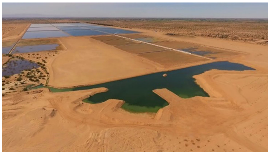
Fig. 8 At San Luis Rio Colorado, Sonora, Mexico, oxidation lagoons (at a wastewater treatment plant in the background), have annually discharged 8.2 \text{ Mm}^3 treated water to intermittent infiltration basins (located at a distance in the middle of the photo) for more than 10 years, and in the foreground some water is starting to be used to
