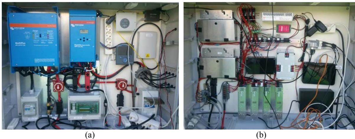
Fig. 9: (a) Inverter, MPPT tracker, protection and monitoring circuit (b) DC-DC converter and protection for DC charging of e-bike
