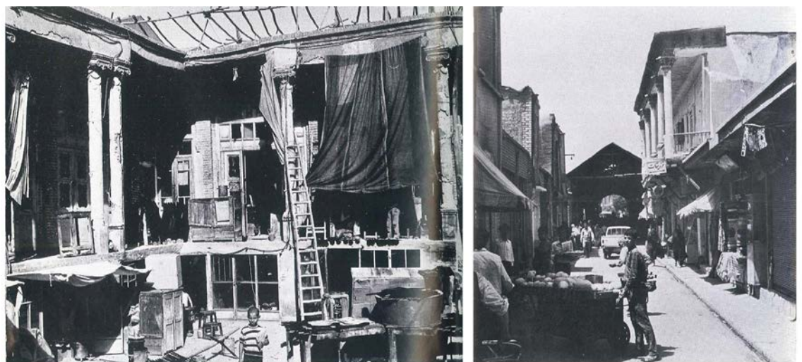
Figure. 4.10. On the left, the condition of housing in historic centre of Tehran. On the right, the back allies of Tehran bazaar.
