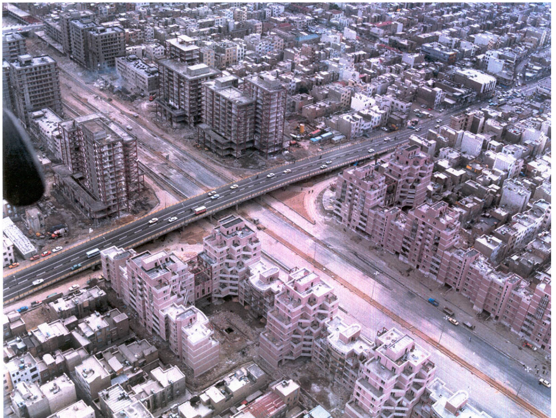
Figure. 5.9. Navab Residential Complex and Highway under construction
