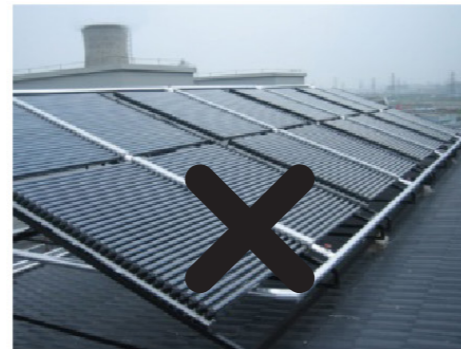
Evacuated tube collectors
