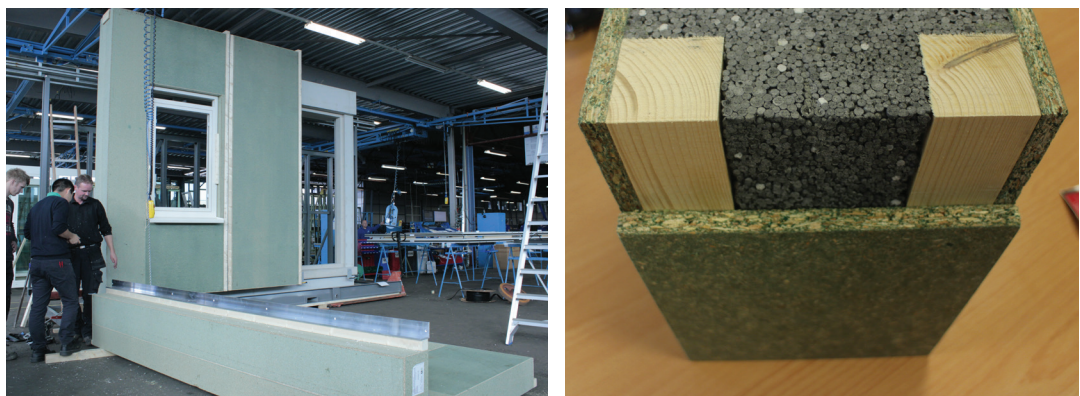
Fig. 30: Photos Mock-up; Left: assembly of SIP-panels Right: section SIP-panel (Konstantinou, n.d.)
