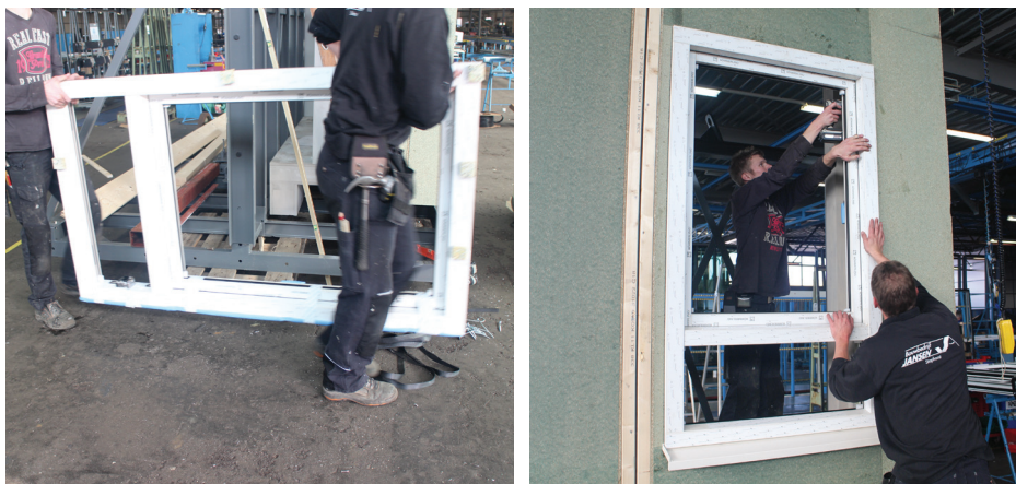
Fig. 31: Photos Mock-up: installation of the K-Vision PVC window frame (Konstantinou, n.d.)
