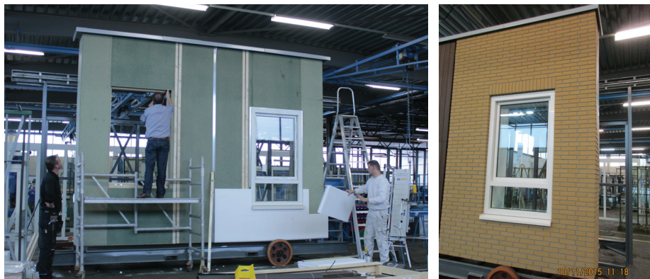
Fig. 32: Photos Mock-Up; StoTherm Classic, brick strips cladding (Konstantinou, n.d.)
