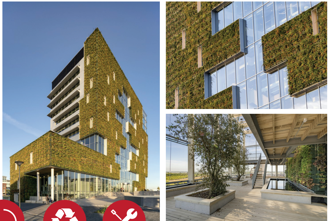
Fig. 14: Photos of the City Hall in Venlo (Kraaijvanger, n.d.)
