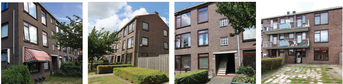
Fig. 25: Photos of the case study building Soendalaan, Vlaardingen (KAW Architecten, 2017)
