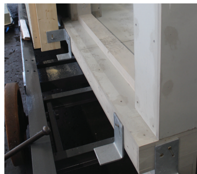
Fig. 29: Photos Mock-Up; connection method substructure (Konstantinou, n.d.)
