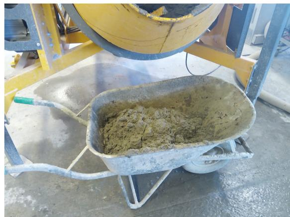
Figure III.3: Mixing step 3: adding cement and water
