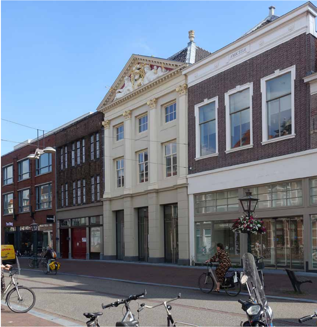
9. PHOTO OF THE CURRENT SITUATION OF THE BREESTRAAT FACADE
