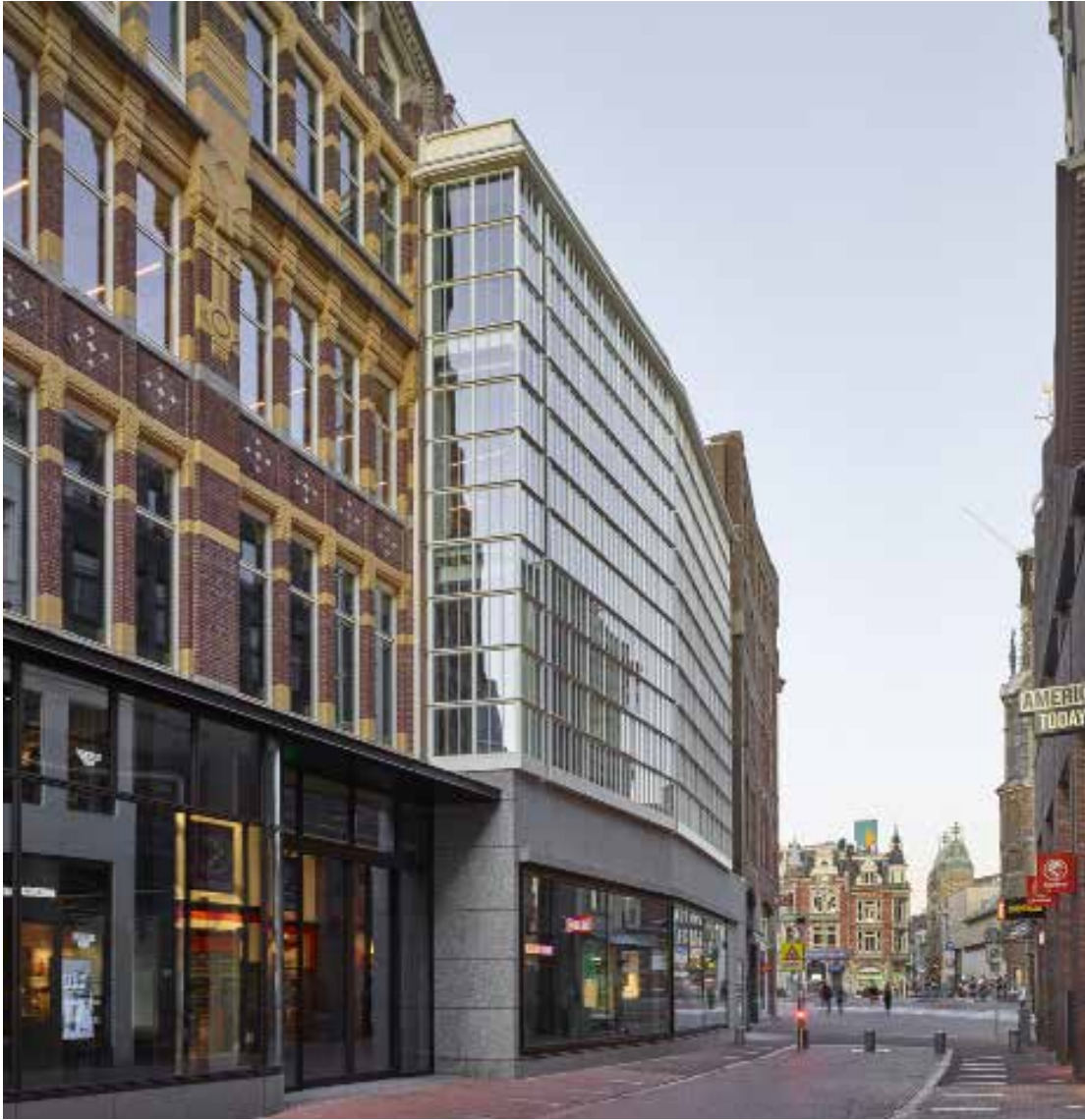
9. PHOTO OF THE CURRENT SITUATION OF THE KALVERSTRAAT FACADE
