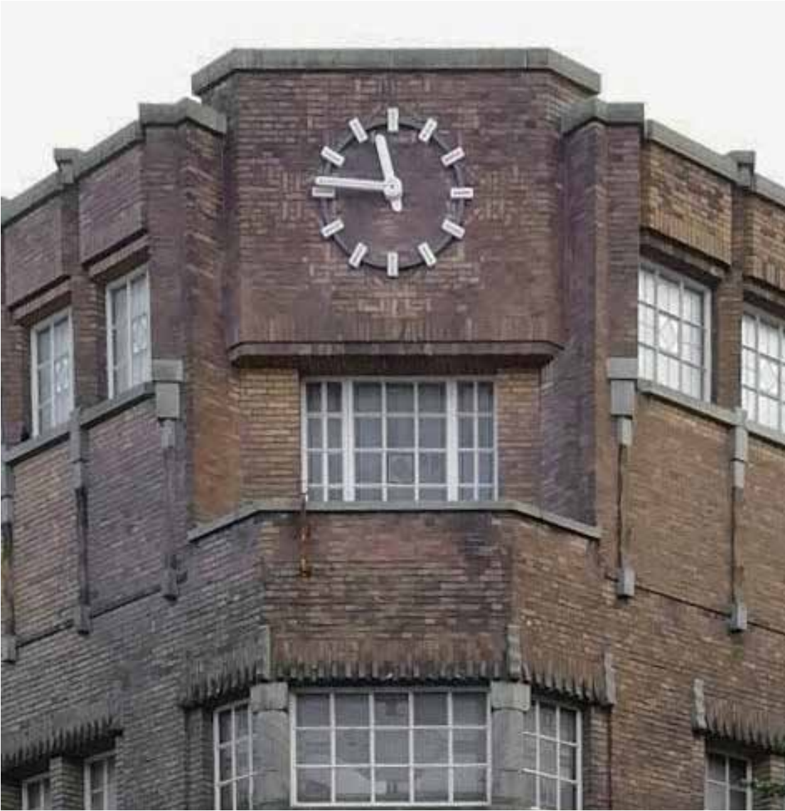
7. FRAGMENT PHOTOGRAPH OF THE LAAT AND RIDDERSTRAAT FACADE
