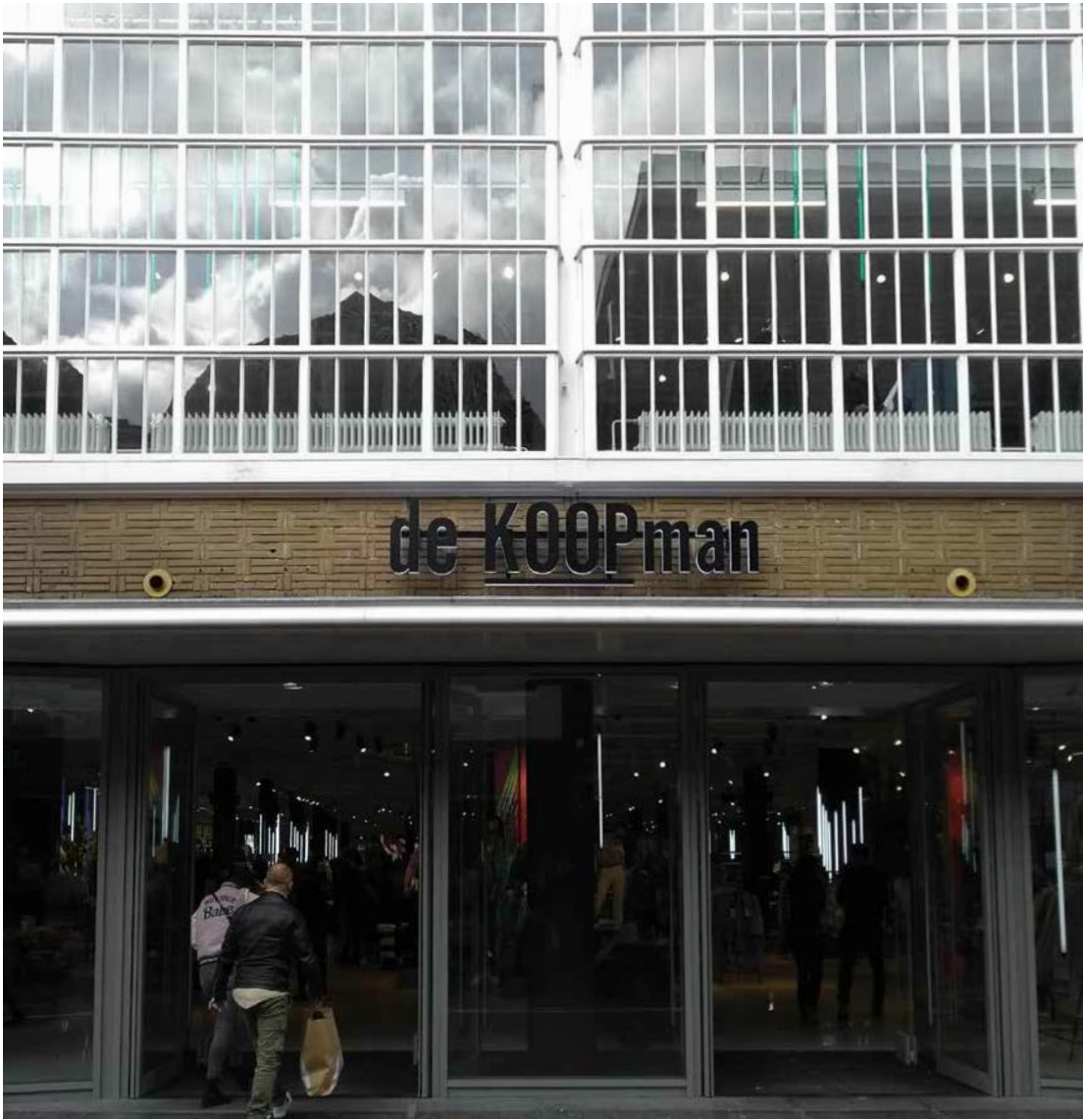
9. PHOTO OF THE CURRENT SITUATION OF THE UTRECHTSESTRAAT FACADE
