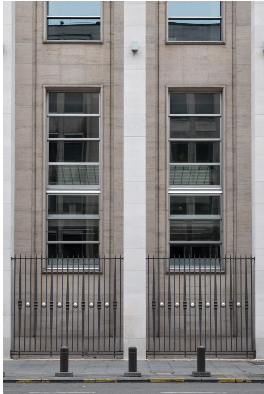
Photograph fragment of main facade
