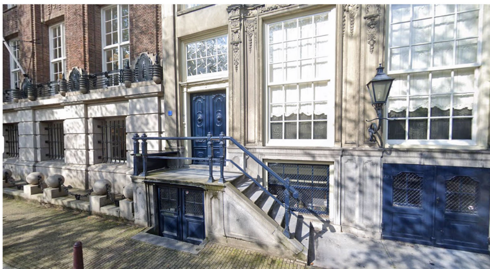
Figure 13. Example of a 'half-floor' for a building in Amsterdam. Notice how the adjacent building does not have this half-floor. Source: Google Street View (2022).
