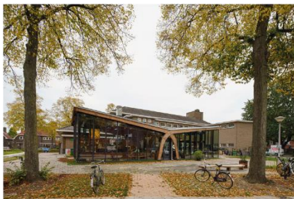
Wooden structure from laminaed timber elements
