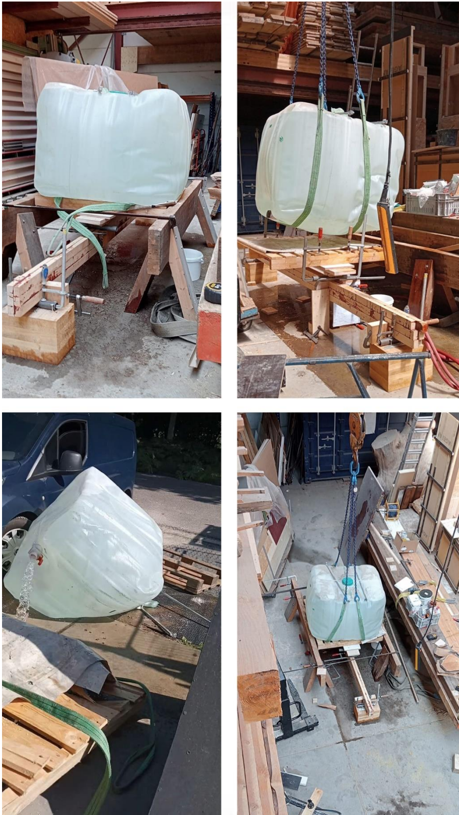
FIGURE 106: USING WATER TANK AS A LOAD (OWN WORK )
