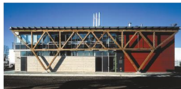
Reusing reclaimed structural truss components
