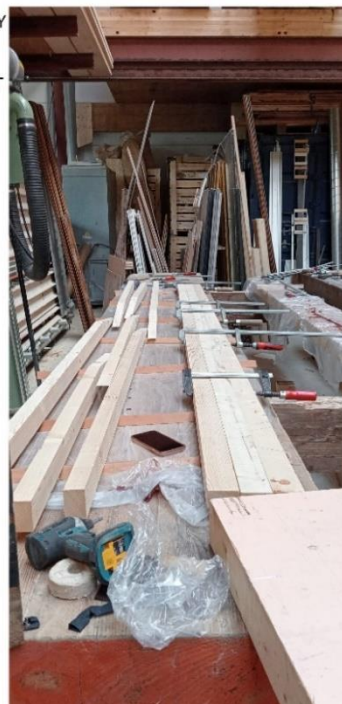
PLACING THE PIECES ON THE WORKING BENCHES AND PLANNING THE THE CUT
