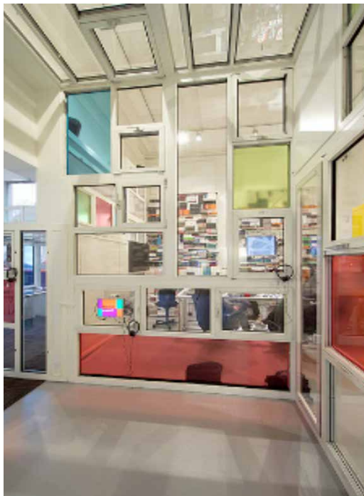
FIGURE 5.5 Internal office partitions made with reused PVC window frames by SuperUse studio ( www.superuse-studio.com ).
