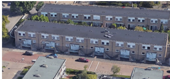
Figure A.17: The example building for determine the energy pattern for buildings of typology 3 built between 1983-1988 (by author and google maps)
