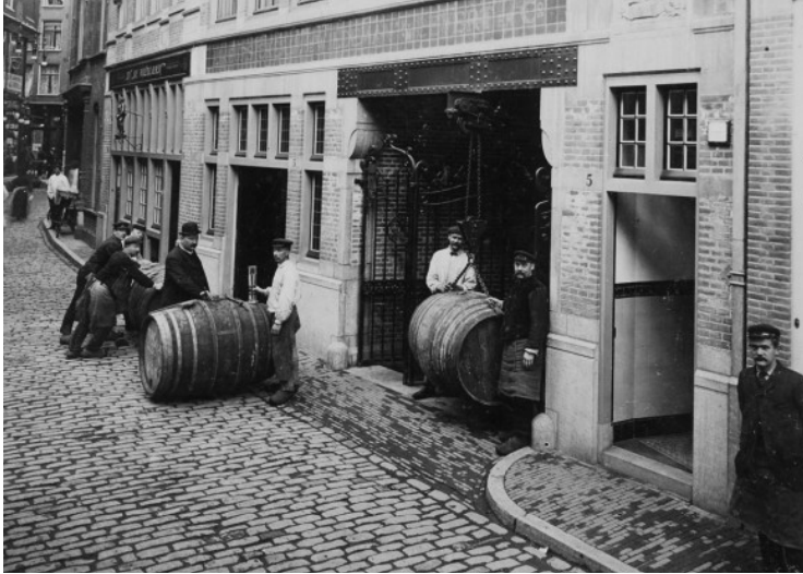
Fabrication activities integrated in the city of Amsterdam.
