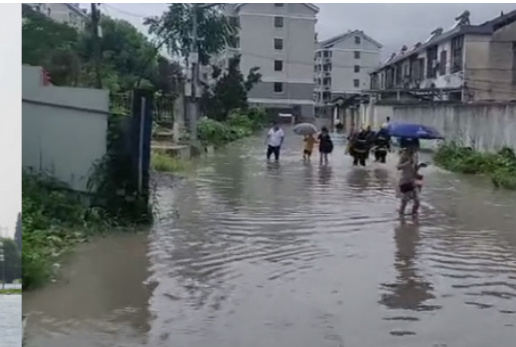
FIG4.8 waterlogging in the city
