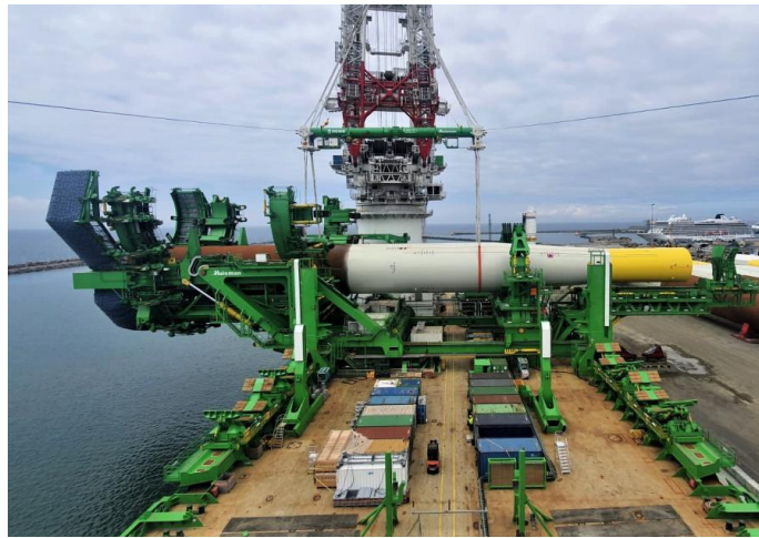
Figure 4.4: Motion compensated monopile gripper frame installed on Orion [32]
