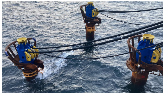
Figure 5.54: Simultaneous drilling operations for the Saint-Brieuc offshore wind farm in 2022[114]
