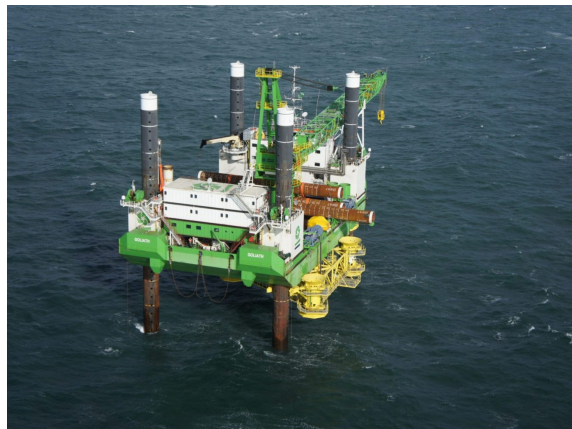
Figure 5.44: Pre piling template hanging under the deck of vessel Goliath [95]
