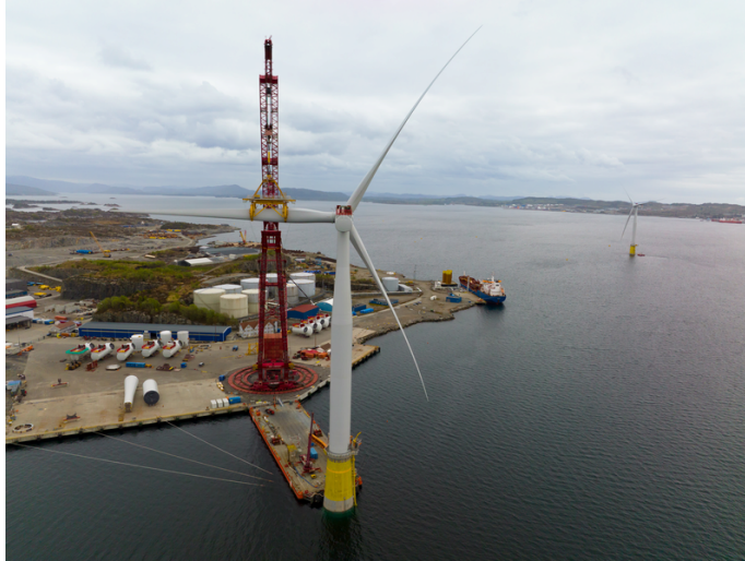
Figure 4.29: Hywind Tampen turbine assembly [71]
