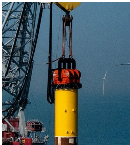
Figure 4.7: CAPE-VLT-640 vibro lifting tool [38]
