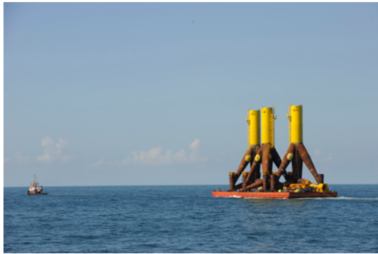
(a) Transportation by barge of three tripod foundations to the offshore installation location [63]
