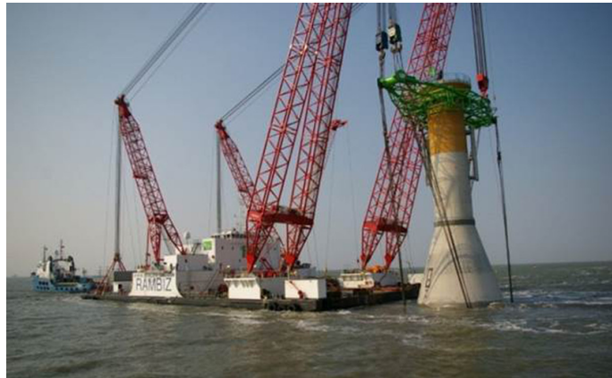
Figure 4.18: Suspended transportation of gravity-based foundation for Thornton Bank wind farm [56]
