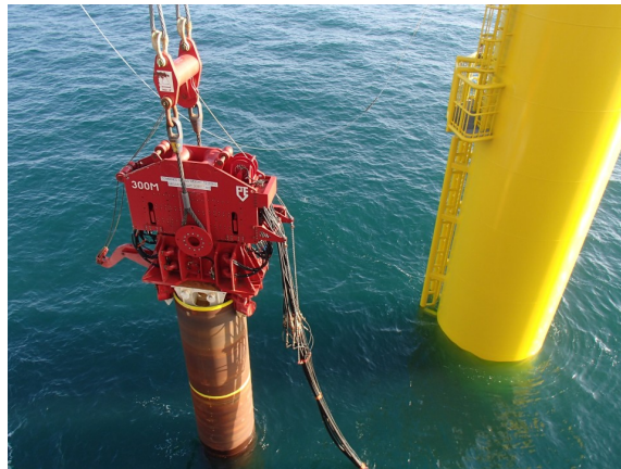
Figure 4.23: Pin pile installation with vibratory hammer for a tripod foundation [65]
