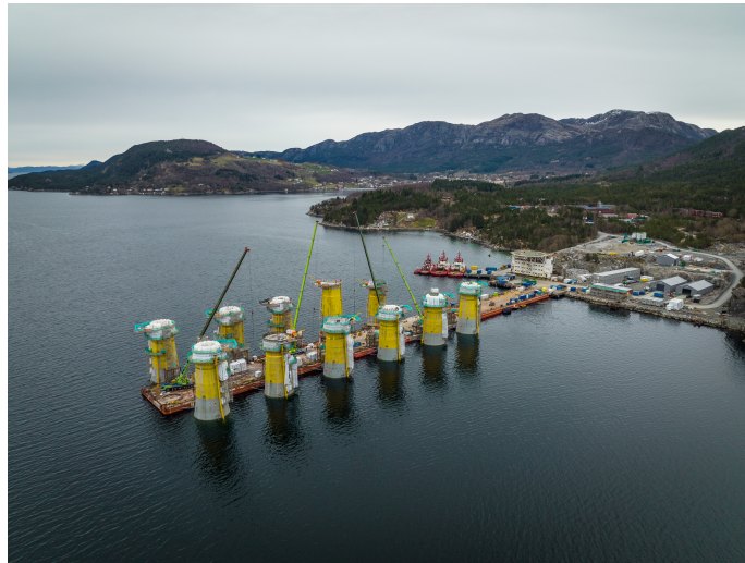
Figure 4.28: Manufacturing of floating foundations for Hywind Tampen offshore wind farm [70]
