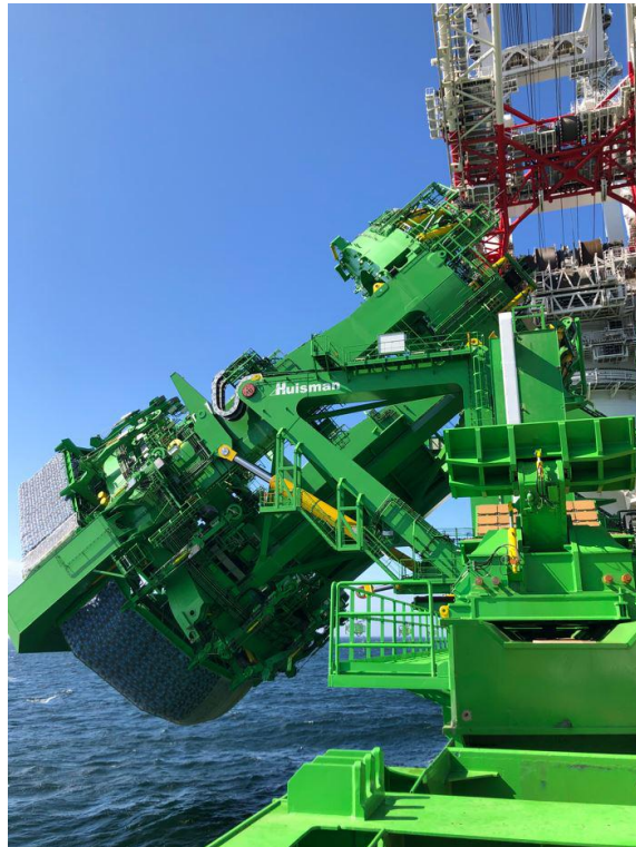
Figure 5.55: Motion compensated pile gripper on the Orion vessel by DEME [119]
