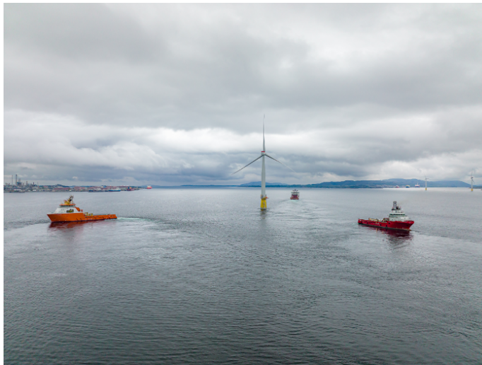
Figure 4.30: Towing of a floating wind turbine to its installation site at Hywind Tampen offshore wind farm [72]
