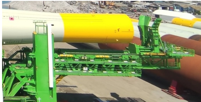
Figure 4.5: Outrigger frame installed on Orion [32]
