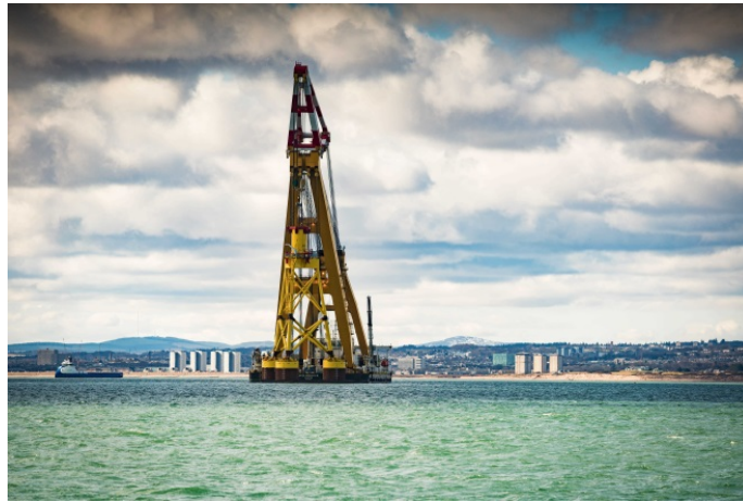
Figure 4.25: Transportation of SBJ foundation for EOWDC wind farm [67]
