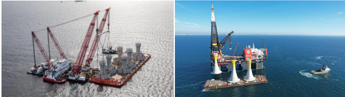
(a) Offshore lifting of gravity-based foundation for Karehamn wind farm from transportation barge by Rambiz vessel [59]
