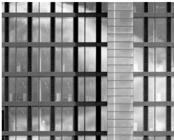
(a) Debitel Headquarters, Stuttgart, RKW Architektur + Städtebau, 2002
